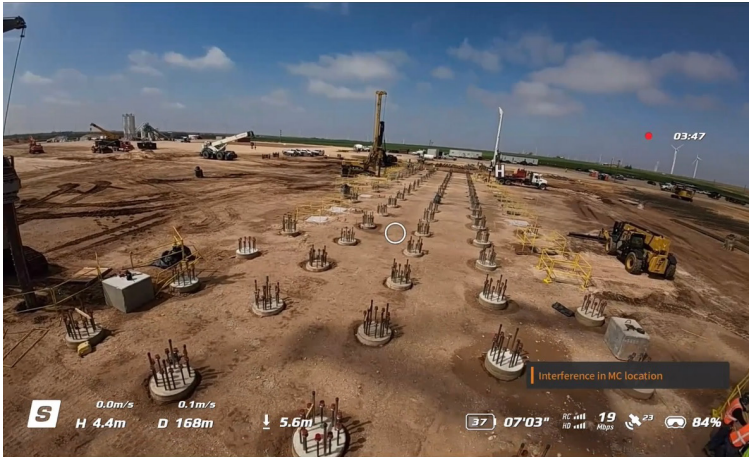
EVx construction Snyder, Texas
